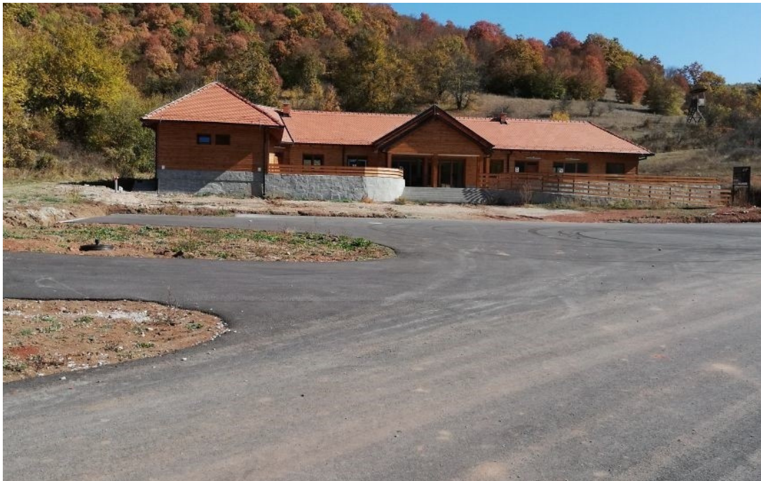
Completed Cerje Road
