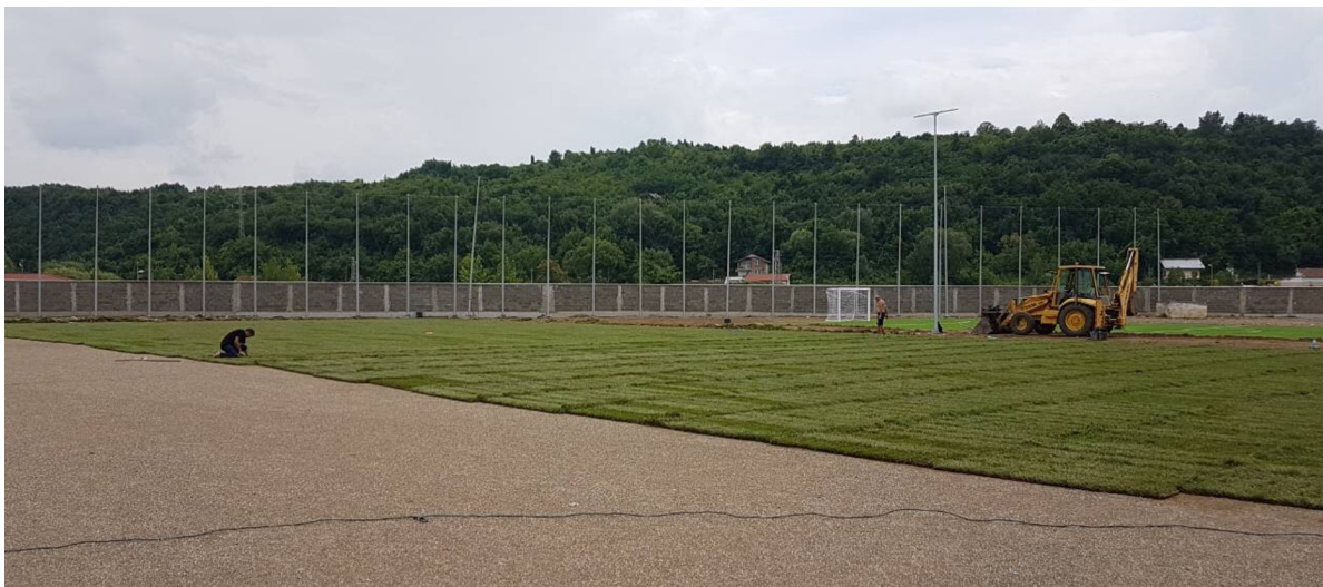
Stadium in Montana, work in progress
